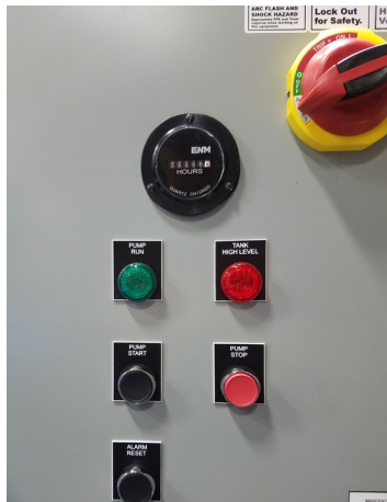
Control panel with hour meter and high-level shut down.
