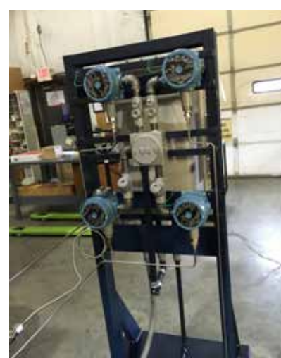
Backside of Nema 7 control panel showing Nema 7 controls which were prewired and connected to compressor and panel.
